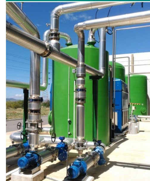
CLAMBER Pilot Plant
